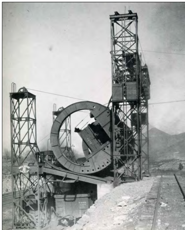
Figure 33. As the junction of standard gauge and narrow gauge lines, Salida housed this barrel transfer structure which inverted narrow gauge gondolas from the upper track into standard gauge ones on the lower track. SOURCE: Thode, George L. Beam and the Denver & Rio Grande , vol. 1 (1986), 137, pre-1957-58 image.
