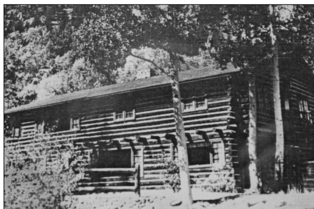
Figure 40. Ray Summe and his sister Ethel Poundstone built this lodge of used telephone poles on South Cottonwood Creek in 1950. SOURCE: Officers Christian Union, brochure, 1963.
